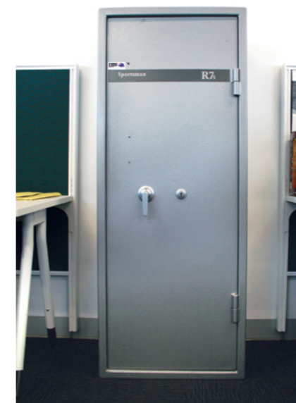
Large safe showing the correct installation method, fixed to the floor and the wall.
